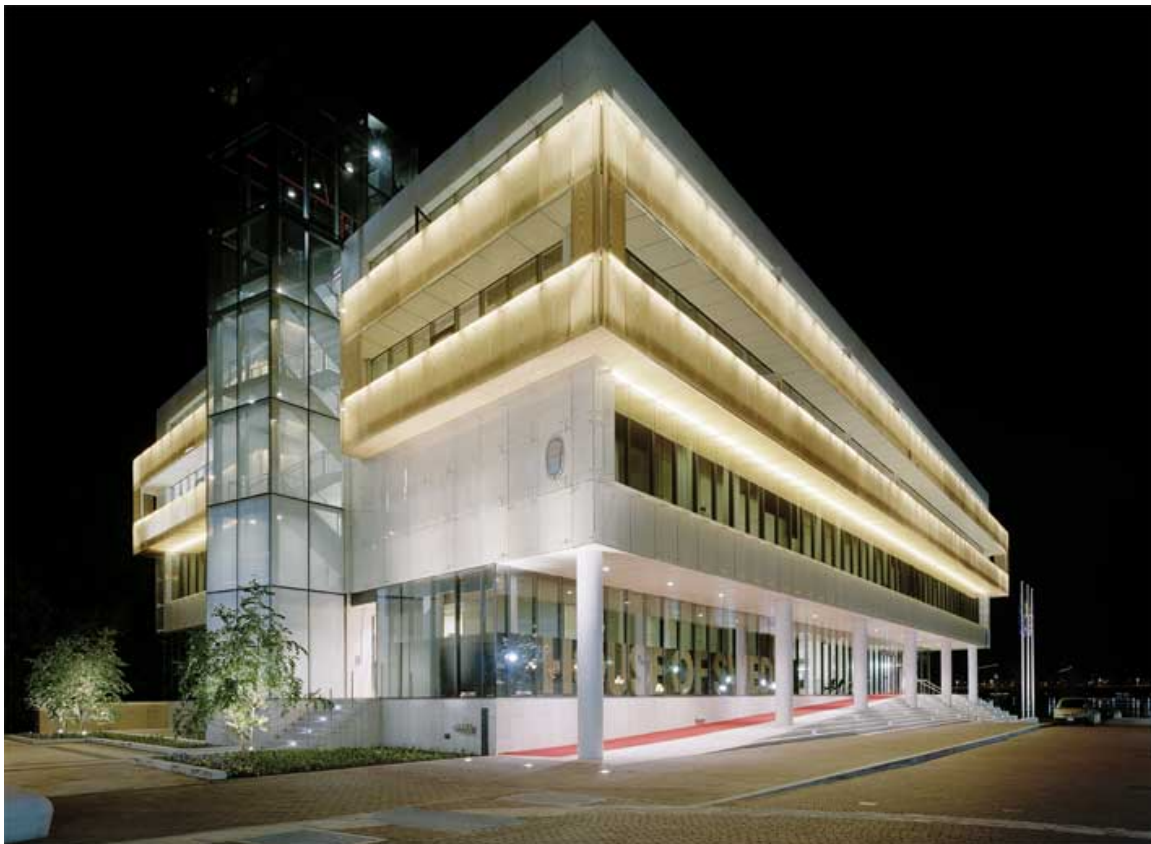
Figure 2A: Night View of the North Building
